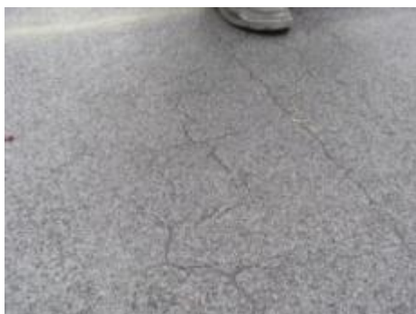
Revner i overpappen
