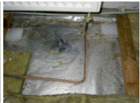
Varmerør under parketgulv
